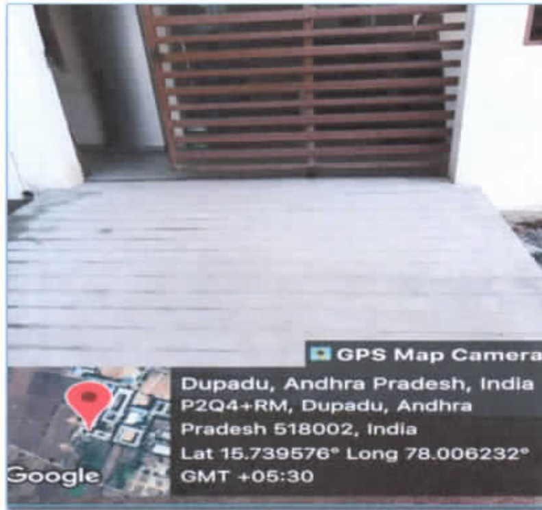
Ramp access into the college
